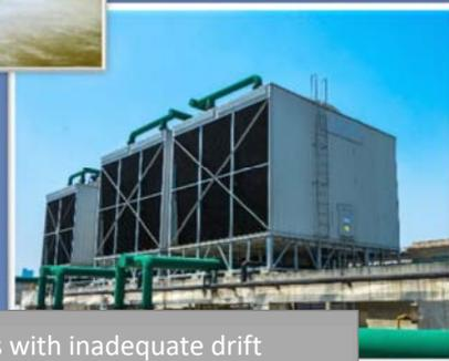
Cooling towers with inadequate drift eliminators can expose passersby to mist.
